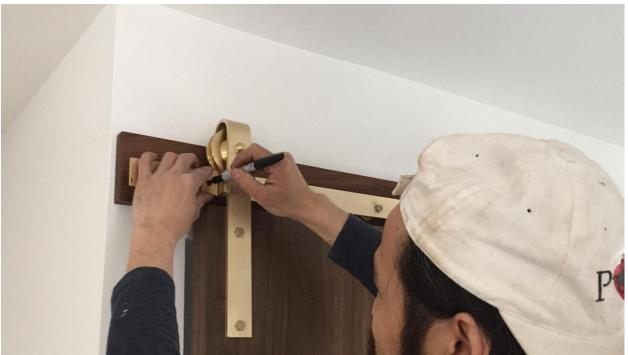
Use 5/16" drill bit to drill holes for stopper. It is a good idea to put a piece of wood behind the track directly behind the hole being drill to prevent drilling into the wood block
