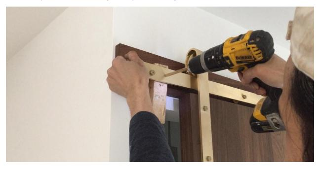
Use provided nuts and bolts to fasten the stoppers to the track.
