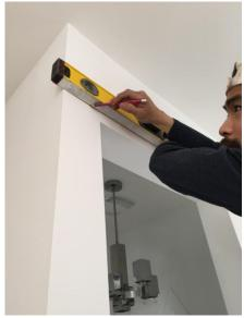
Use 3" long size 8 construction screws (not provided) to fasten the wood block to the wall studs. 2 screws are recommended for every stud. Test for level.
