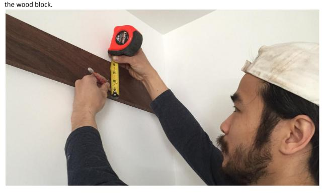
Lay the track on the wood block and mark the drilled holes onto the wood block. Make sure the track is leveled.
