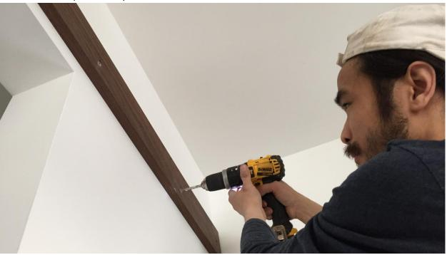
Use provided 5/16" x 4" lag bolts and spacers to fasten the track to the wood block. Note, the flanges on the spacers are to face the wood block. Check for level and adjust if necessary.
