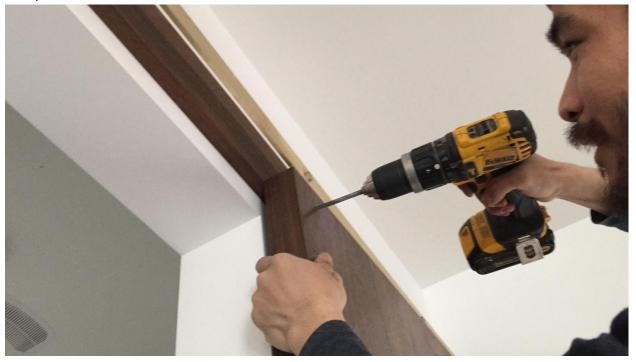
Use provided 5/16" x 1.5" lag bolts to fasten the hangers on the door.
