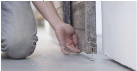
Guide for the outer door will be install on the front of the inner door, closer to the edge in the direction where the door travel to close.
