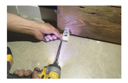
Install bottom stopper plate on inner door
