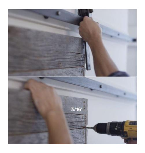
Use provided 5/16" x 1.5" to fasten the hangers onto the door. Repeat for the other inner hanger.
